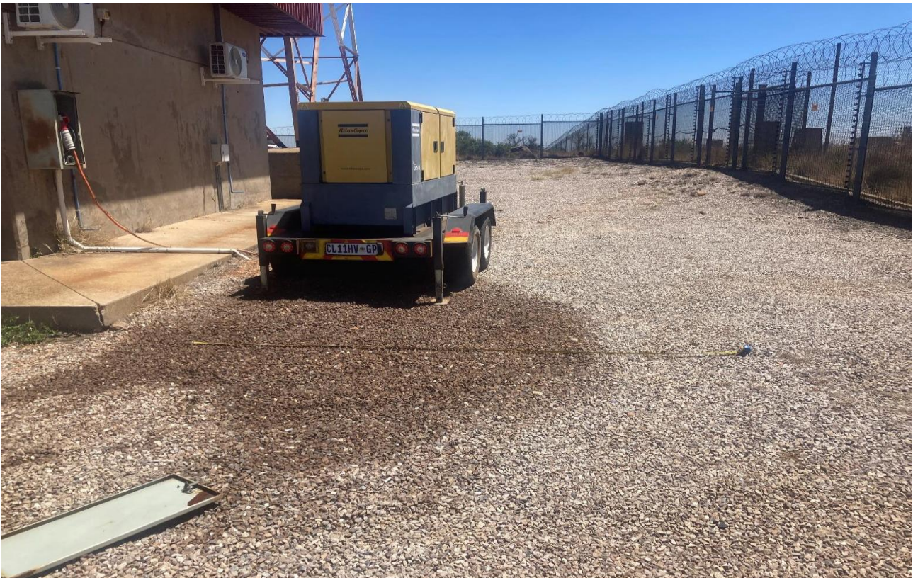
Figure 1: Mobile Generator positioned in the selected position for new generator plinth and shelter
